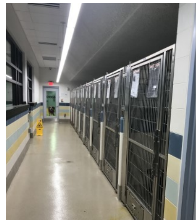
Figure 2 - Urine in walkway during hours open to public at 11:10 am on January 24, 2020.
